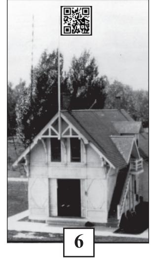
The main section of the Life Saving Station housed the wagon that carried the life saving equipment. It was dispatched to aid ships wrecked in the water. A Lyle gun shot a lifeline over the ships rigging so as to pull a heavy duty "Zip line" from shore. The harness was a pair of "breeches" attached to a life ring for survivors to climb into.
